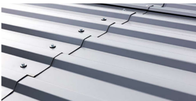
EXTRUDED METAL ROOF WITH EXPOSED HARDWARE
