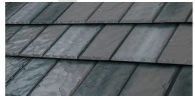
SLATE METAL ROOF
