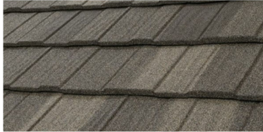
SHAKE METAL ROOF
