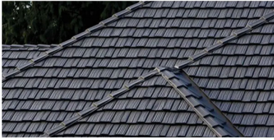
STAMPED METAL ROOF
