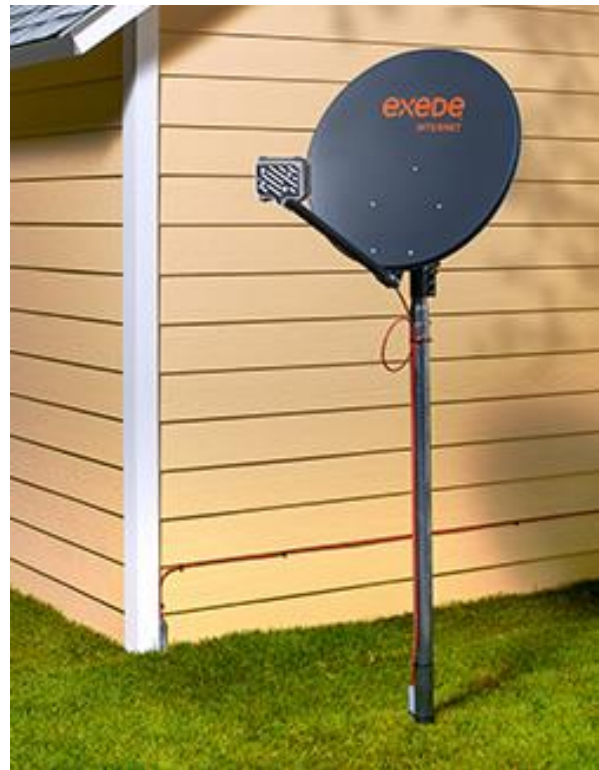
FIGURE 2. Acceptable pole mounted dish antenna
